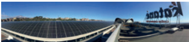
Catania_Katanè_ Photovoltaic system
