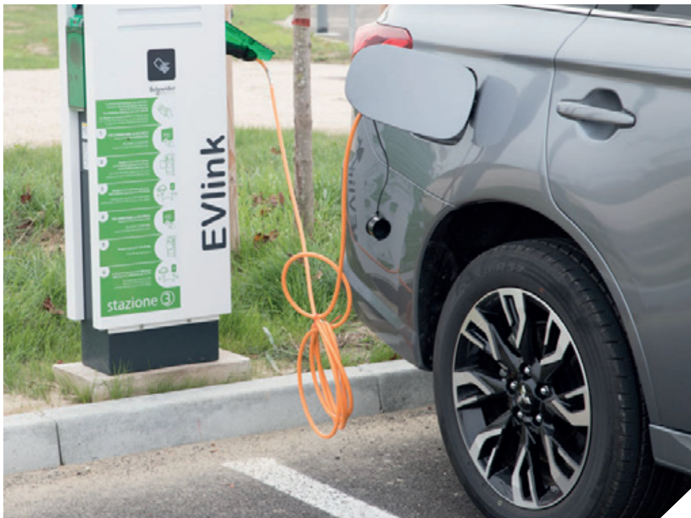
Ravenna_ESP_EV charging station
