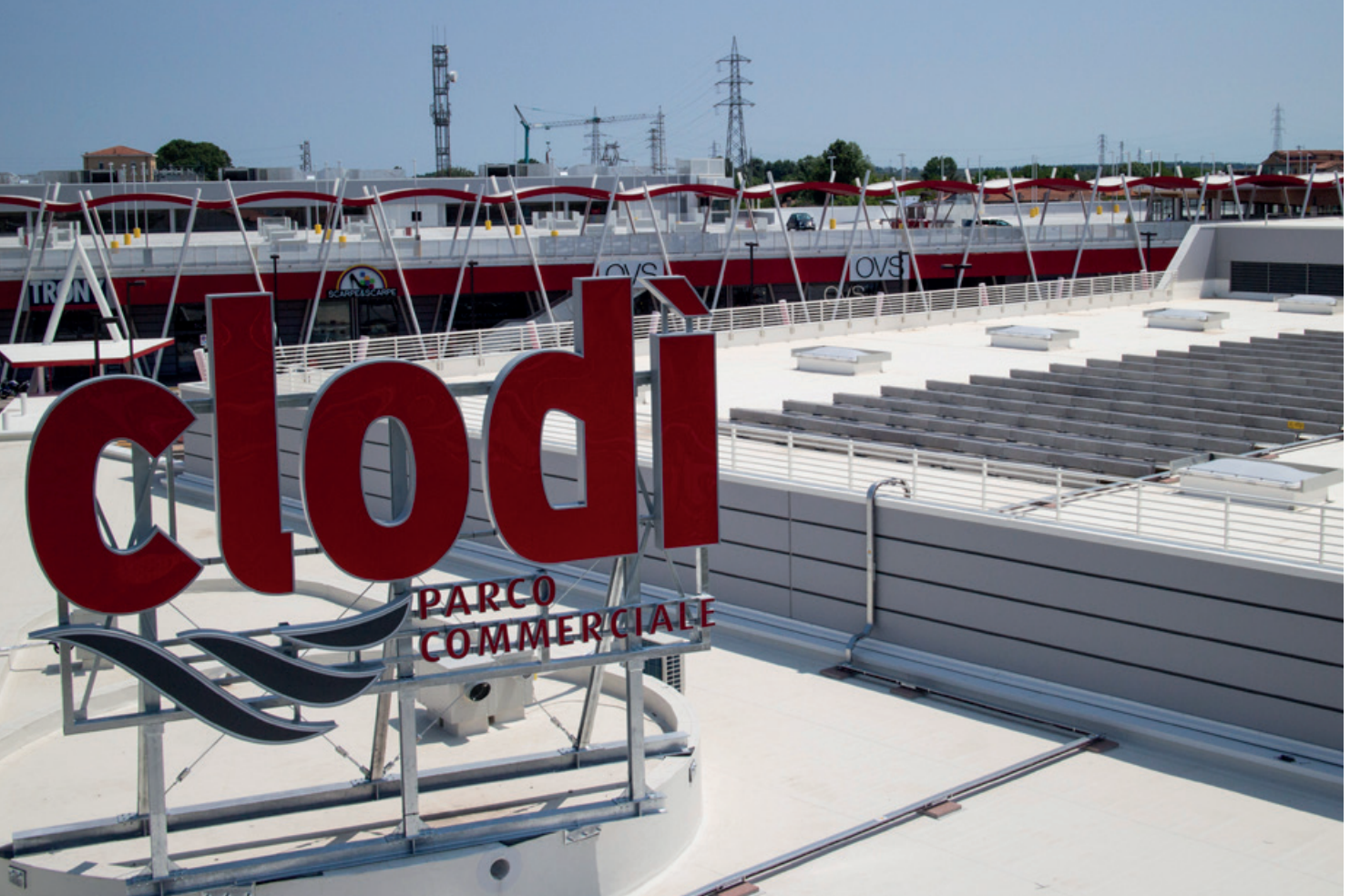
Chioggia (Venice) Clodi Photovoltaic system
