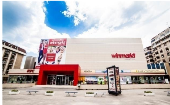
Ploiesti Omnia: facade restyling nearly completed
