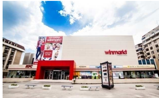
Ploiesti Omnia: facade restyling nearly completed
