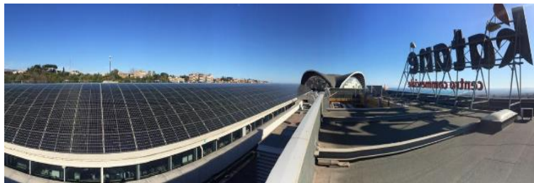
New photovoltaic system in Katanè
