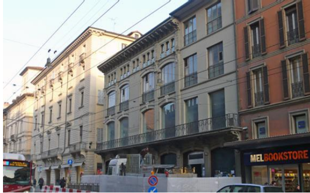
Before the beginning of the works
