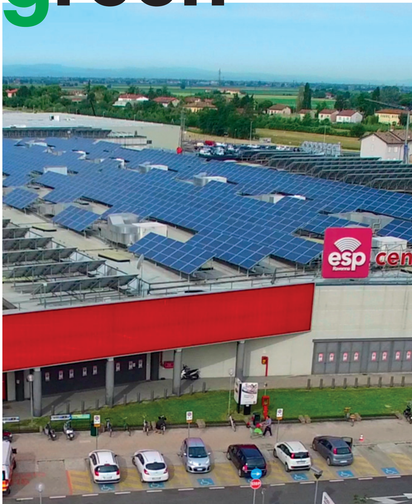
Ravenna ESP_Photovoltaic system
