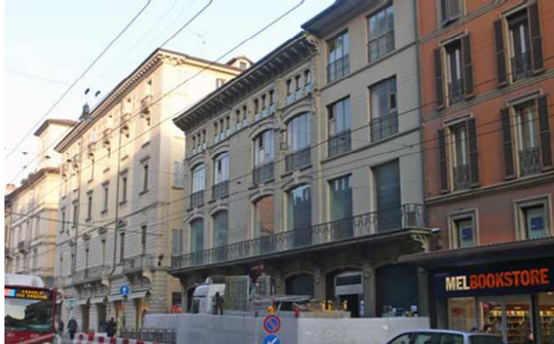
Before the beginning of the works
